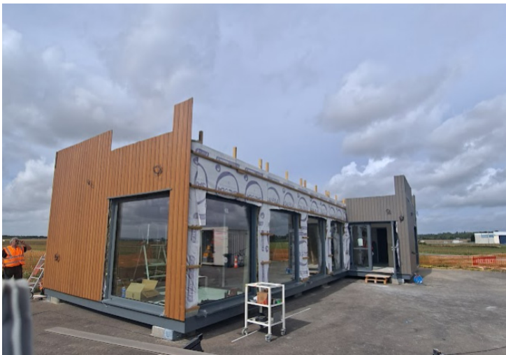
Figure 9 Vertiport under construction – IPAX
