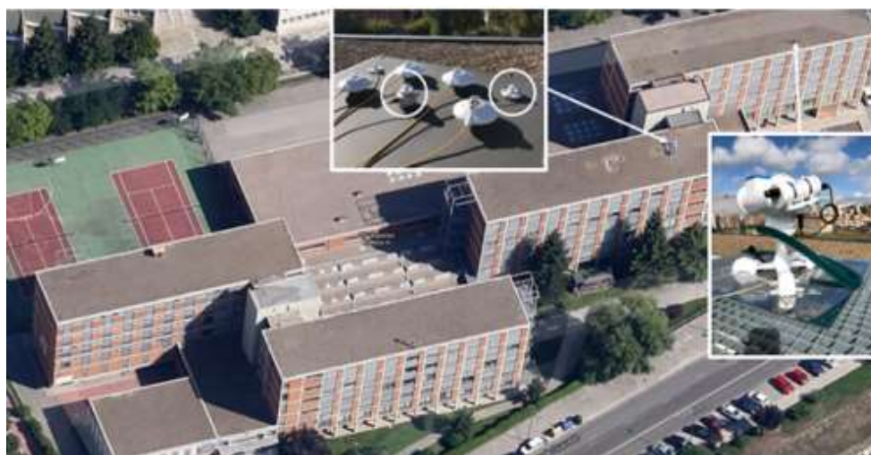
Figure 2. Location of the experimental equipment on the roof of the Higher Polytechnic School building at University of Burgos, Spain.
